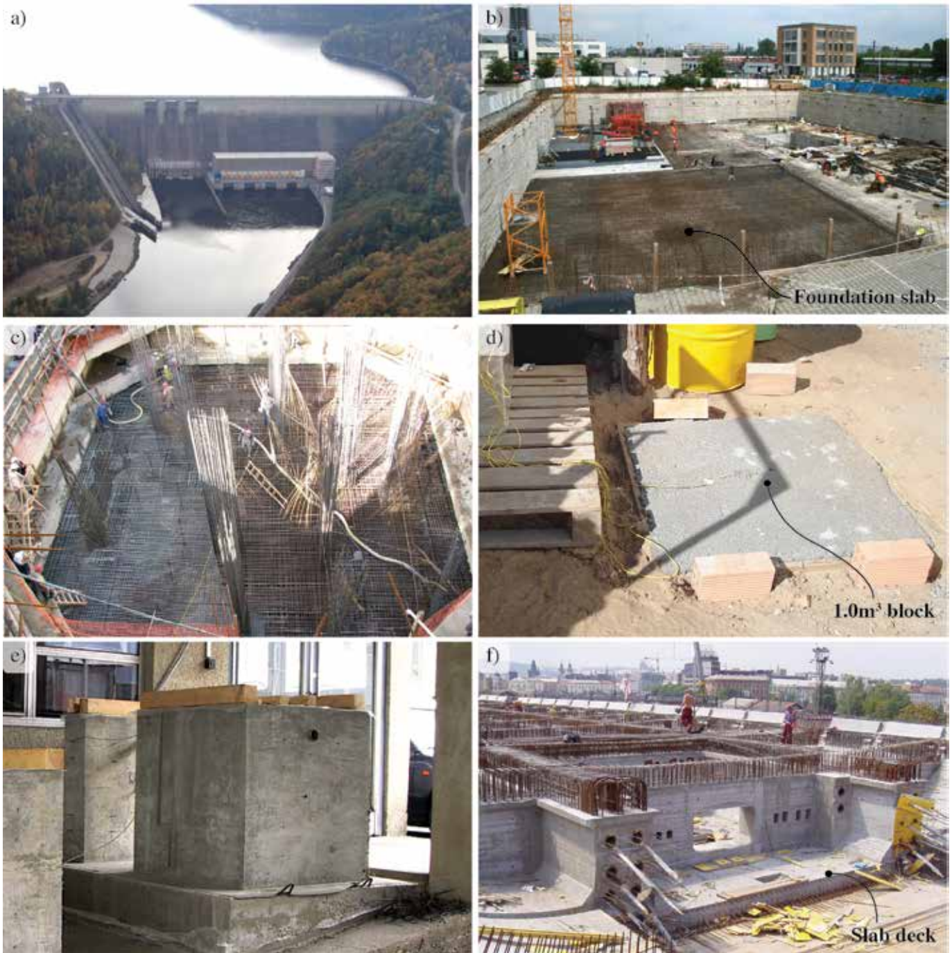
Fig. 7: Investigated mass concrete structures: (a) V1: Orlik Dam, Czech Republic; (b) V2: Foundation slab, AZ Tower, Brno, Czech Republic (photo courtesy of R. Hela); (c) V3: 1050\text{ m}^3 ( 37,065\text{ ft}^3 ) foundation block, Torre d'Napoli, Balneario Camboriú, SC, Brazil (photo courtesy of Formula F10 Empreendimentos); (d) V4: 1.0\text{ m}^3 ( 35.3\text{ ft}^3 ) concrete block A, Federal University of Santa Catarina, Florianópolis, SC, Brazil; (e) V5: 1.0\text{ m}^3 ( 35.3\text{ ft}^3 ) concrete block B, Czech Technical University in Prague, Prague, Czech Republic; and (f) V6: Bridge slab, Nové Spojení, Prague, Czech Republic (photo courtesy of D. Prause)
